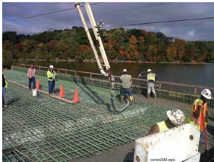
Figure 77 Use of cones can assist with identifying the danger zone
